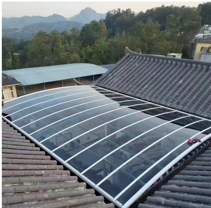
countryard daylighting (clear)
