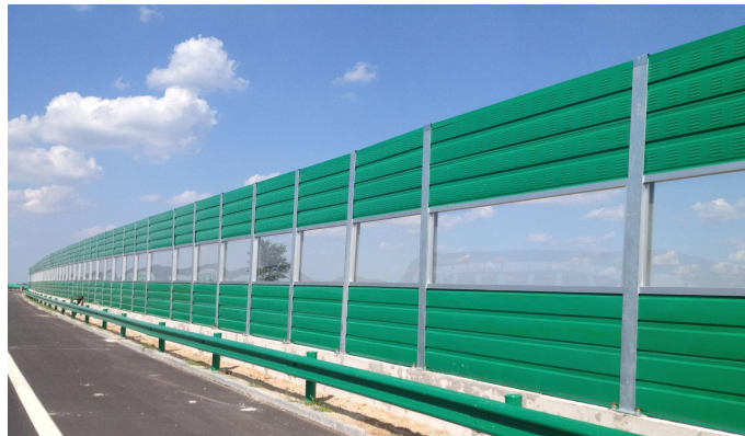
Railroad noise barrier
